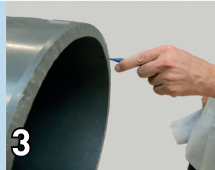
3 Remove internal burrs
