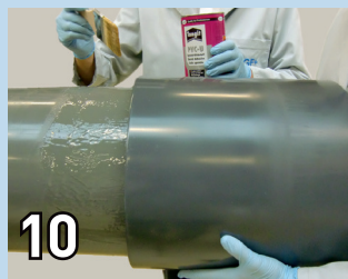
10 Pipe and fitting should be joined slowly and in correct alignment & restrained for at least 1 min (3 to 4 people)
