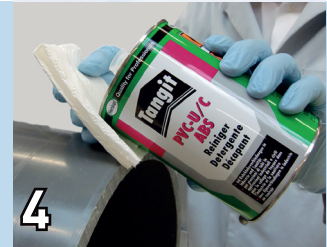
4 Clean pipe and fitting socket thoroughly with TANGIT cleaner & make a fingernail check to examine adhesion (poss. roughen pipe surface)
