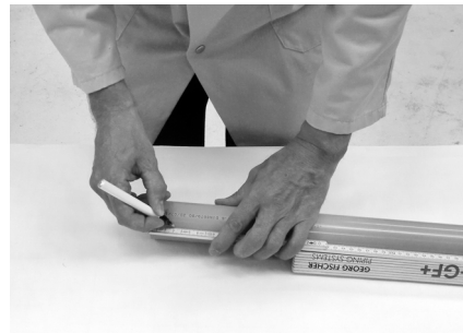
Marking the jointing length
