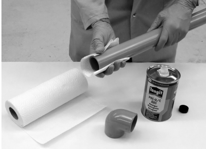
Cleaning the pipe and socket
