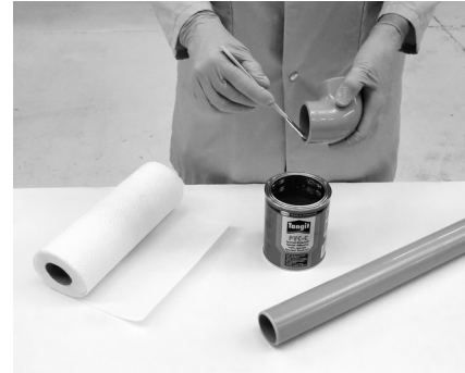
Applying the cement
