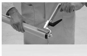
Chamfering the pipe
