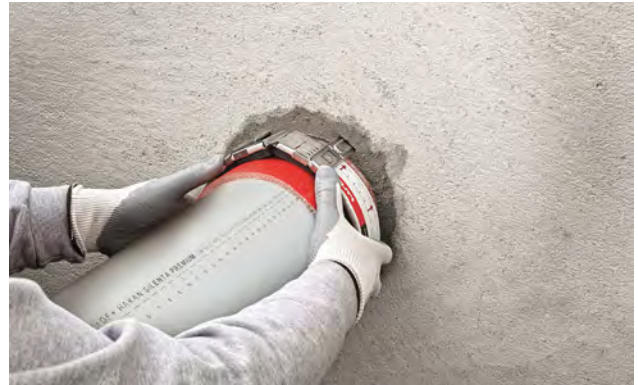
Installation with mortared-in mounting hooks
