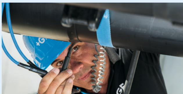
Connect the welding cables to the welding contacts of the fitting and weld according to the instruction manual.
